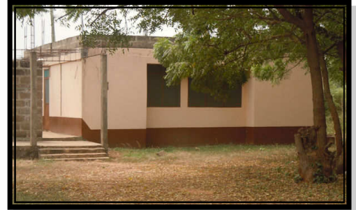
The half-completed duplex
